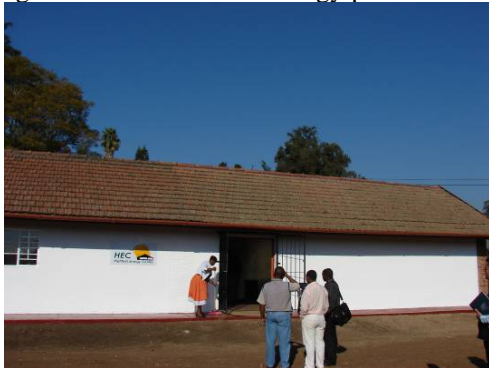
The building housing the Highflats Energy Centre
